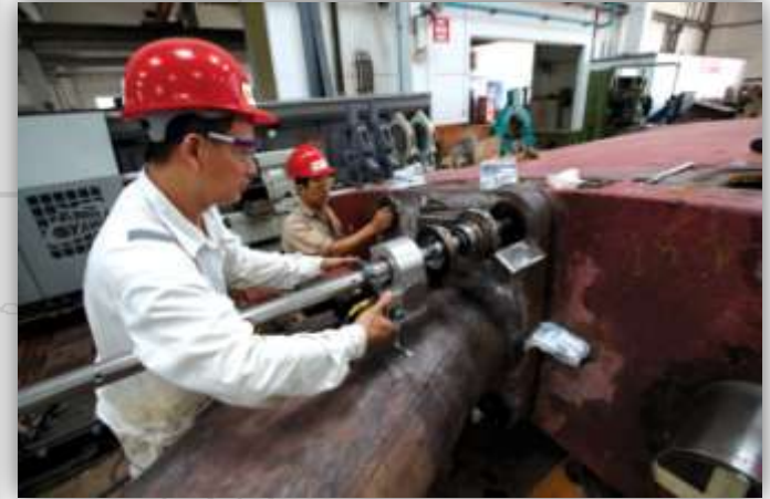
Insitu-boring of Fit Bolt Holes
